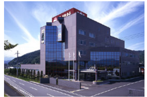
Hokuseisha's main plant: integrated production from planning to printing and publishing
